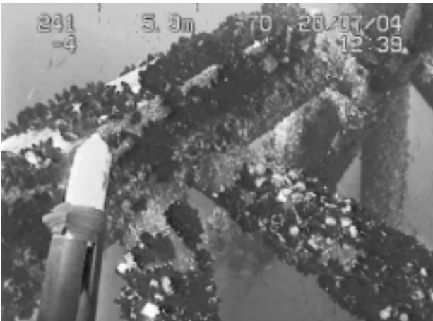
Figure 8: Underwater inspection of structural elements 8 Slika 8: Podvodni pregled strukturnih elementov
