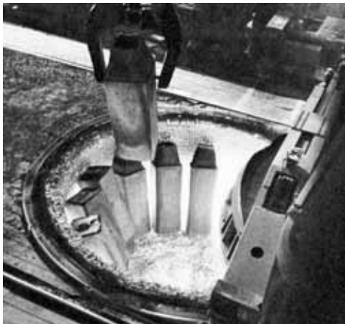
Figure 9: Charging of ingots in the pit furnace Slika 9: Zakladanje ingotov v talno peč
