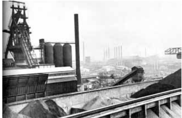
Figure 6: Ore bedding with a view of the blast furnaces
