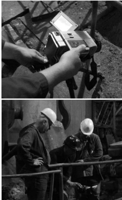
Figure 3: View of the workers making the thermography measurements
