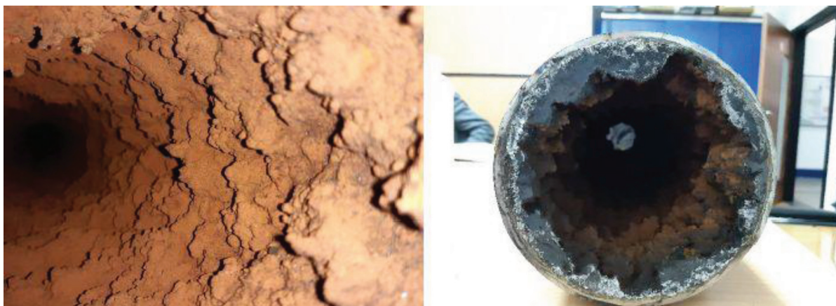
Figure 1: Appearance of the interior of the investigated steel pressure pipeline
